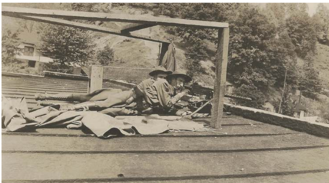
National Guard troops atop a commissary. Note the framework for wet weather tarps.
